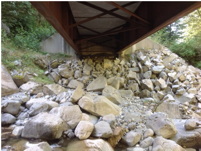
Left Bank Abutment when facing downstream
