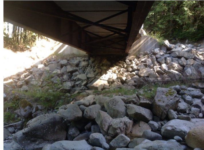
Right Bank Abutment when facing downstream
